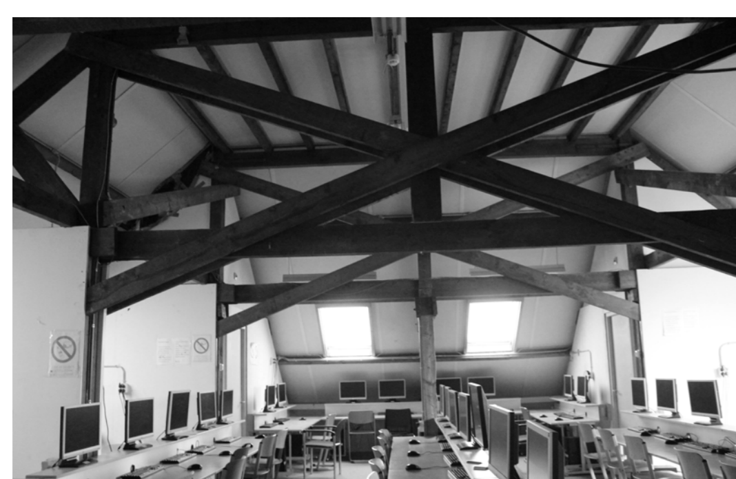
Timber roof construction
